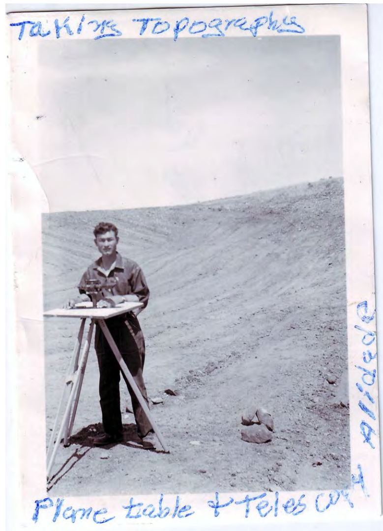
Elson Alvarez surveying with plane table and telescoping
