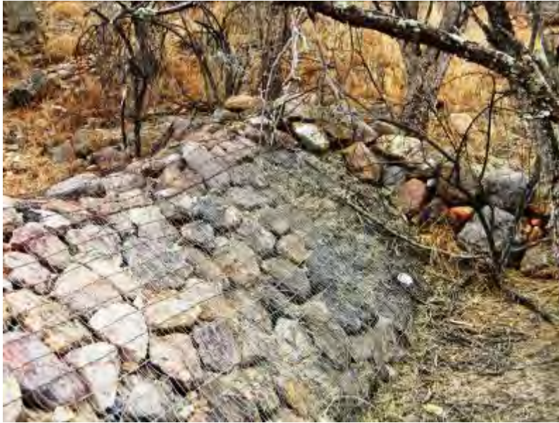
The west end of the gabion abuts the canyon wall. Courtesy Murphy Musick.
