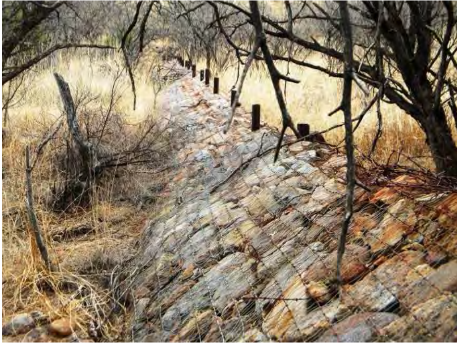
150-foot-long dry-stacked gabion dam in School Canyon, Patagonia, anchored by railroad rails and heavy wire. This dam connects with the earthen dam on p. 111. Courtesy Murphy Musick.
