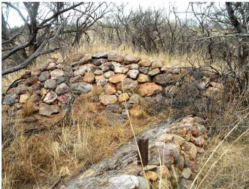
The east end of the gabion dam abuts the west end of the earthen dam. Courtesy Murphy Musick.
